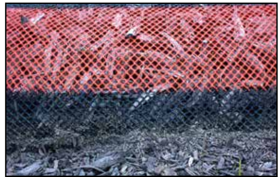
Close Up of Sediment Control
